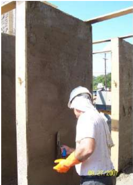
Figure 6: Smoothing out mortar after spraying
