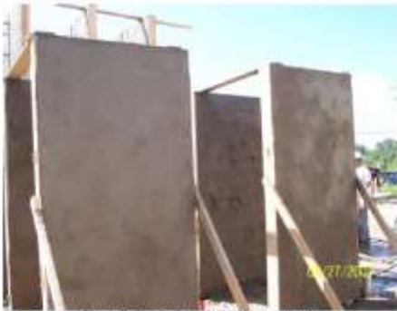
Figure 7: Finished 4' x 8' PSM50 wall panels
